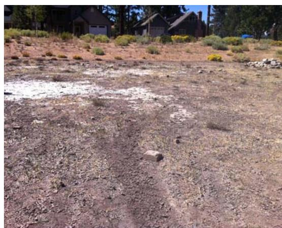
*Layer of fine material accumulation in upper cell of PA2 following sustained inundation in Spring WY11.*
