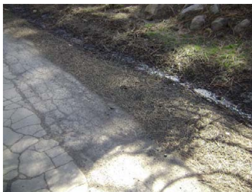
Primary flow path inaccessible to road sweeping or snow haul
