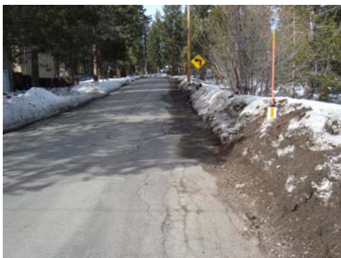
Snow plow disturbance on an unprotected road shoulder
